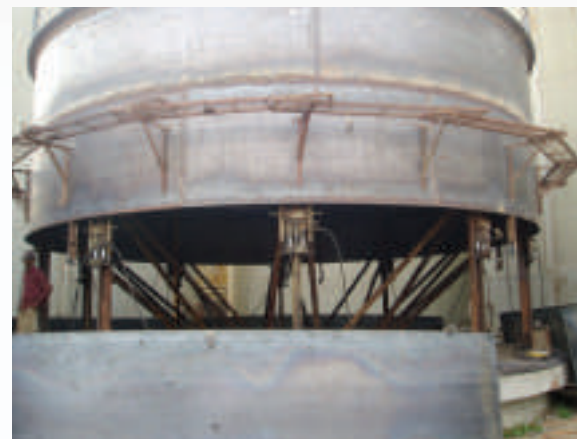
Tank Fabrication by Jacking Method
